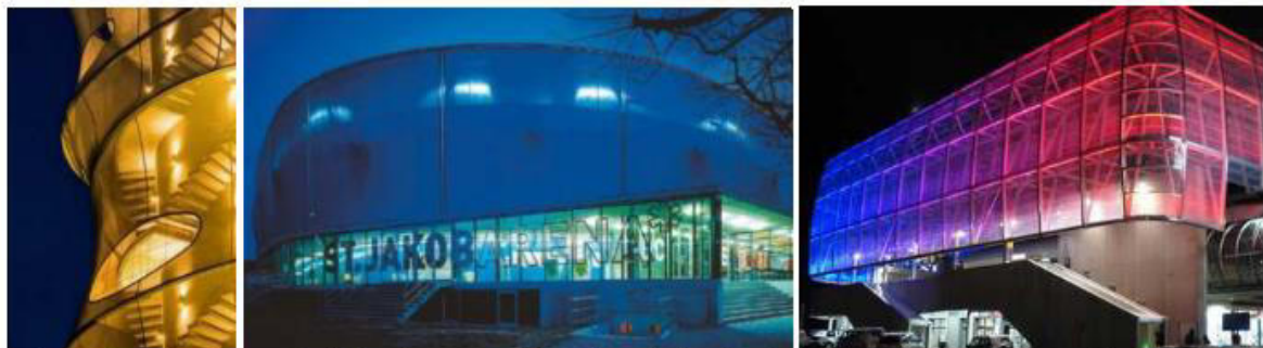
Figure : Sculpture shaped volume of building is more original than during the day by means of transparent skin. Atypical membrane form stand out better without advertising, revealing load - bearing building construction
