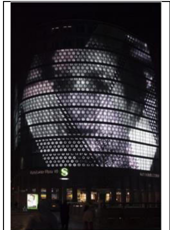
Fig(18) : Media facade
