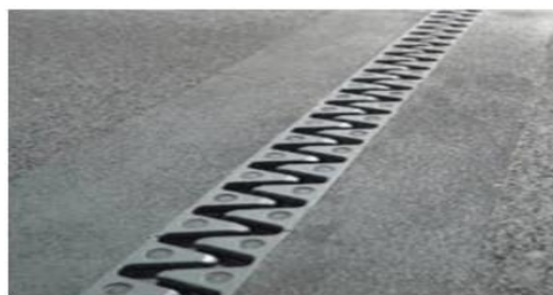
Figure 57: joint de chaussée FT150-Freyssine
