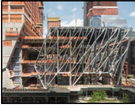
Figure 54 The sliding shell structure "source:(www.archdaily.com;2021)
