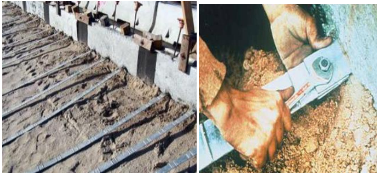
Figure 1.14 Metal reinforcing bars.
