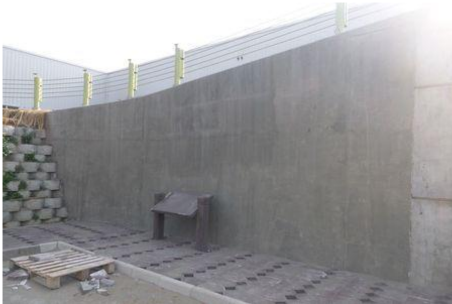
Figure 1.11 Example of Cast-in-place Concrete.
