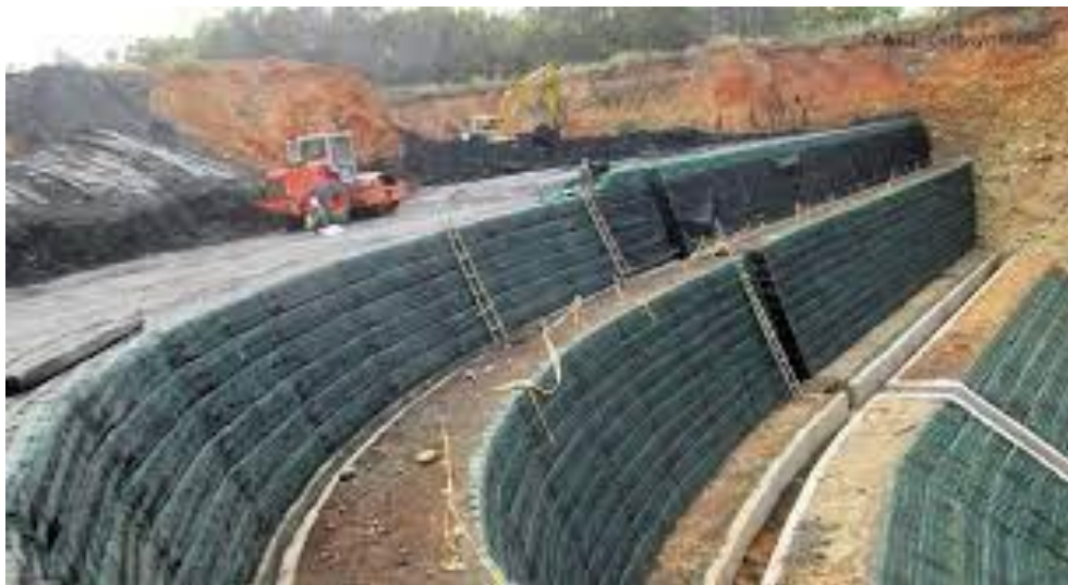
Figure 1.8 Wrap-Around Reinforced Retaining Wall for Collapsed Slope
