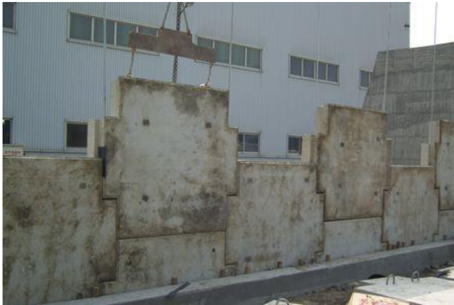
Figure 1.5 Examples of cruciform facing panels.
