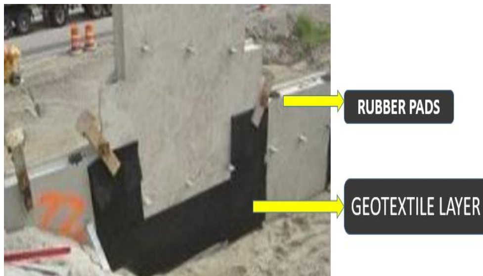
Figure 1.17 Example jointing materials for MSE walls ( https://vincivilworld.com ).
