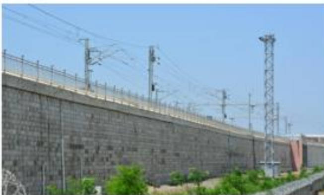
(a) Left side of the GRS wall
