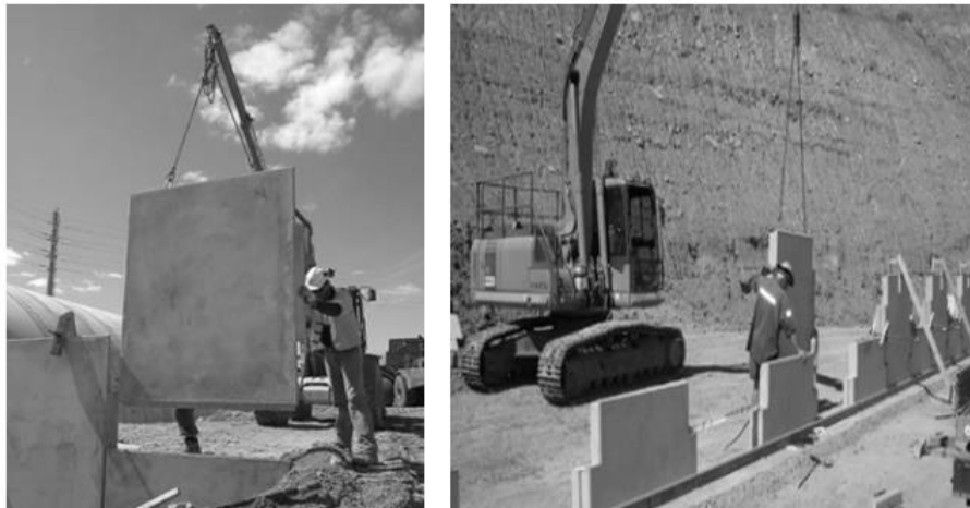
Figure 1.5. Installation and pose the concrete panels (Soletanche Freyssinet ©)
