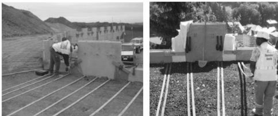
Figure 1.6. Installation of the reinforcements (Soletanche Freyssinet ©)
