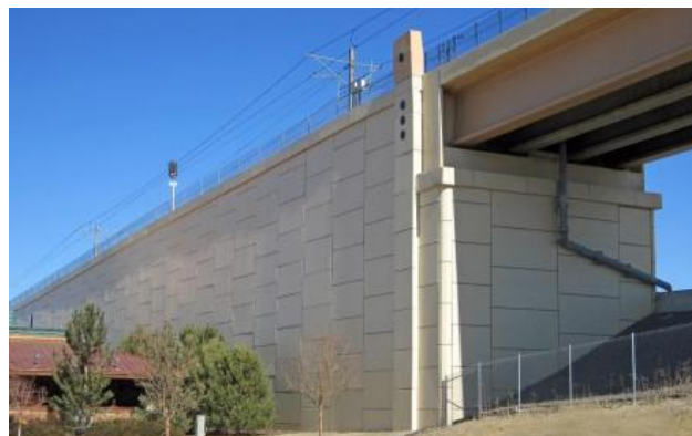
Figure 2.2. T-Rex Rapid Transit, Denver, CO H = 14.0 m, W = 10.1 m, L = 9.8 m, W/H=0.72 and L/H = 0.7 (Anderson et al 2018)
