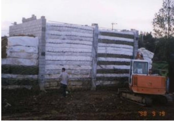
Figure 2.18. The geosynthetic reinforced soil (GRS) walls of Won and Kim 2007.
