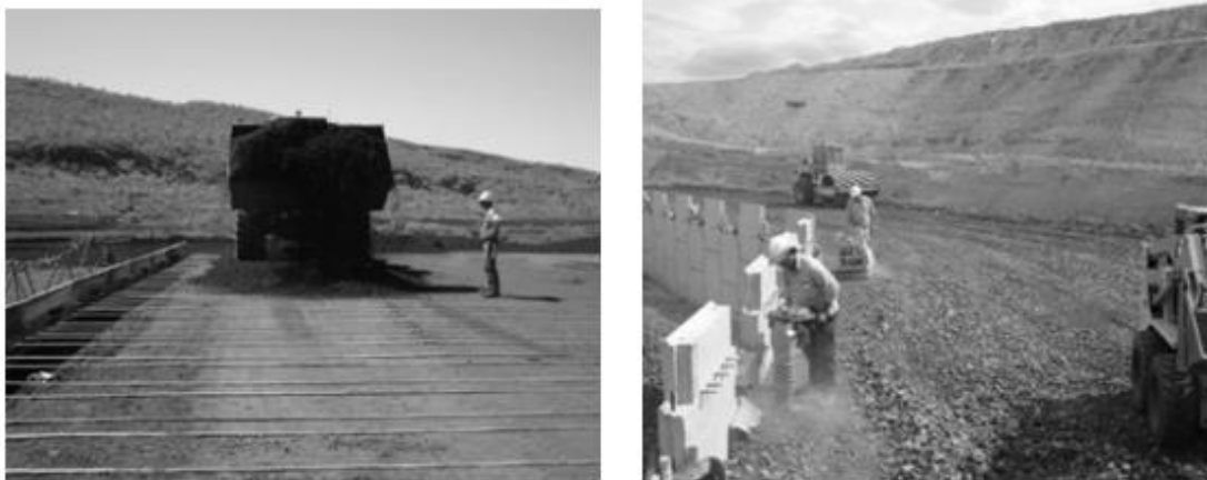
Figure 1.7. Backfilling and compacting (Soletanche Freyssinet ©)
