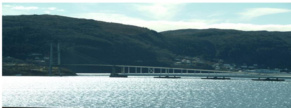
Figure (II.6) : Pont flottant Pountons [97].
