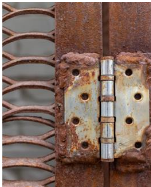
Figure I. 1: corroded hinge [2].
