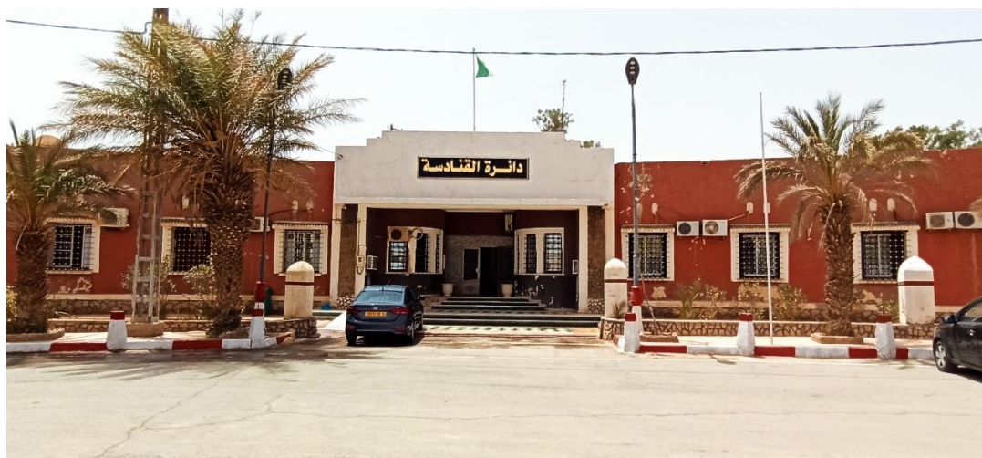
Fig 54- Kenadsa's heritage administrative office building, (author 2024).
